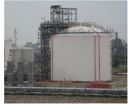
Vopak ammonia tank in Singapore
